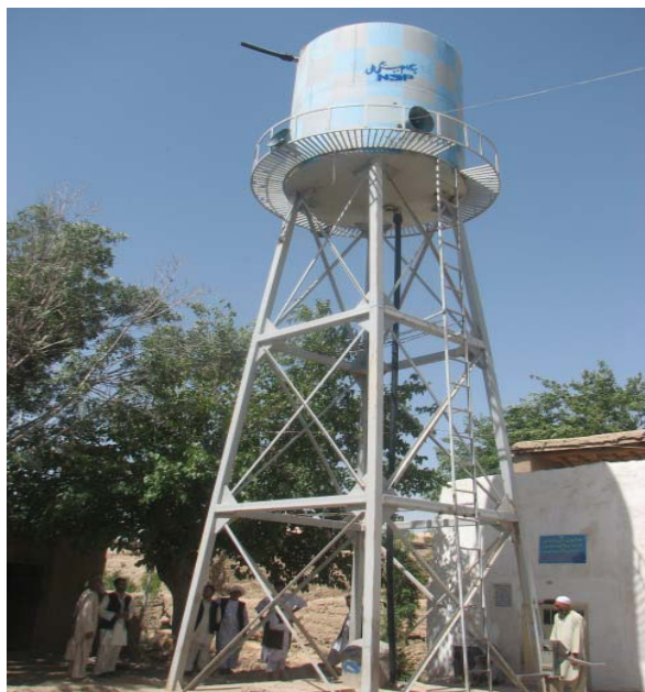
A water tank and water supply network have been established under the National Solidarity Program in Rahman village in Kapisa Province.
