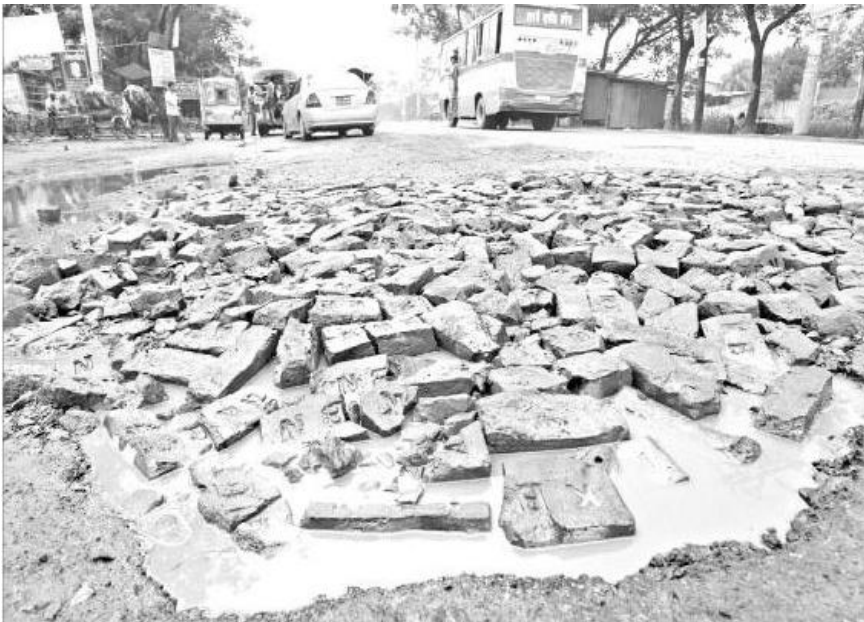
Fixing Roads in a Hurry
