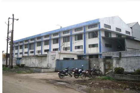
Plant buildings with gates and guard post
