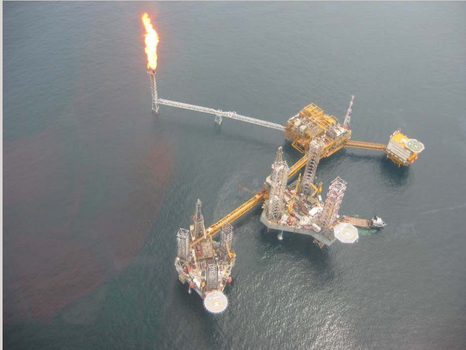
Exxon-Mobil Amenam Platform, Nigeria
