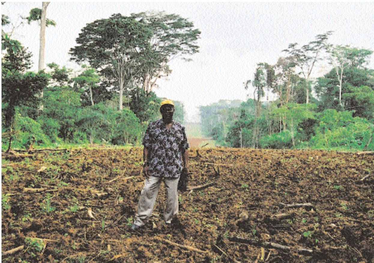
Cameroon: The Pipeline Project—Panel Chairman standing in the middle of the pipeline corridor near Yaoundé.
