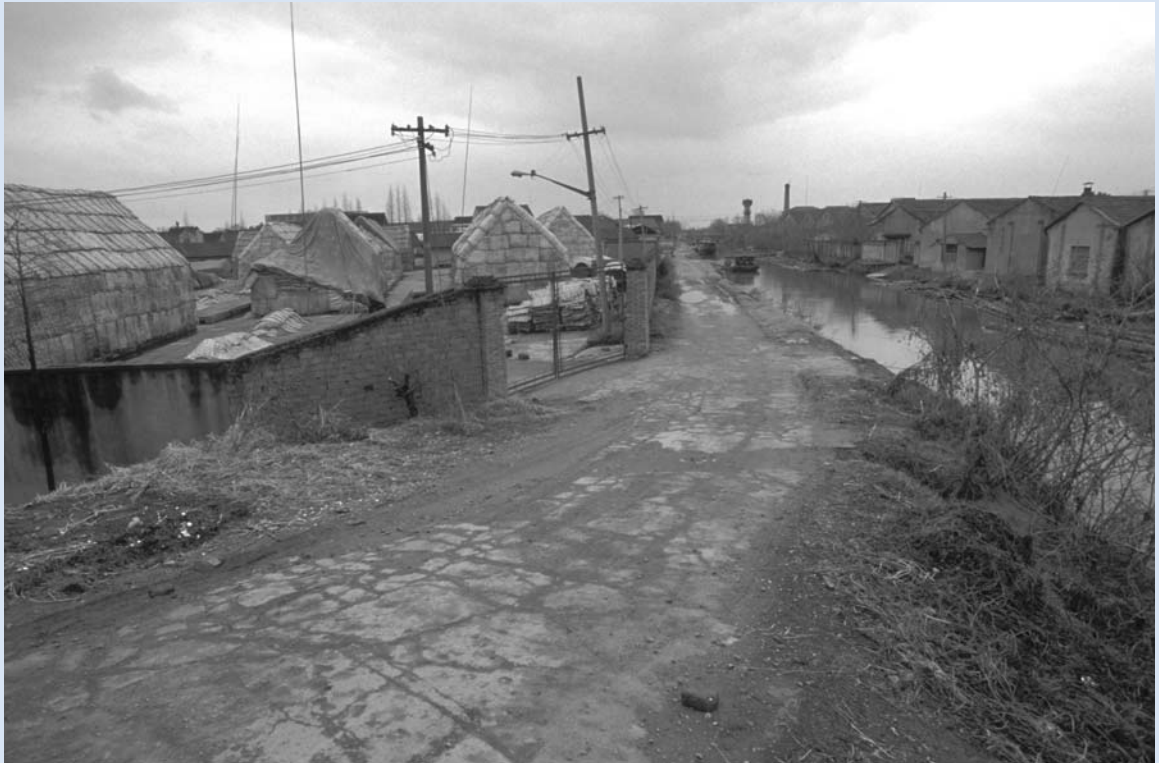
Rural Chinese village with electric poles. (Photo from the World Bank Photo Library.)
