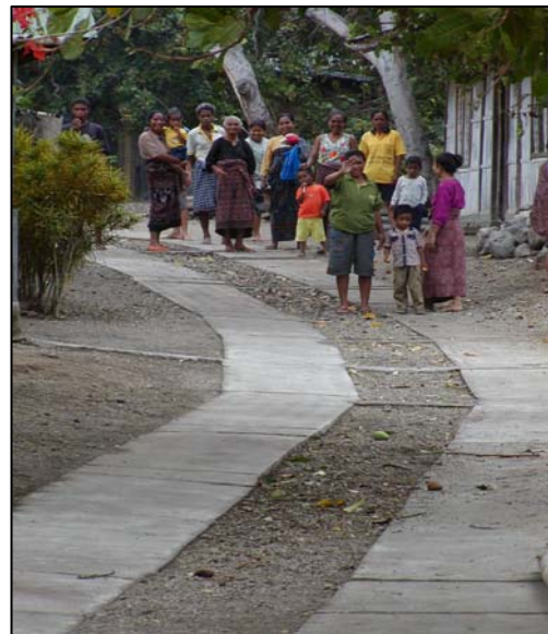
Villagers at a KDP rural road construction project
