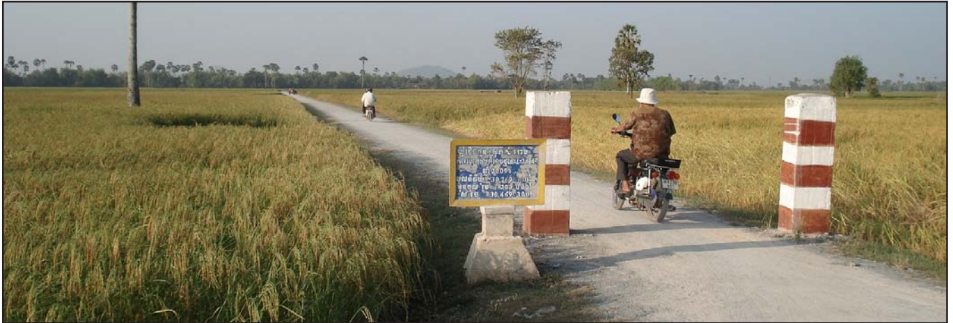
This 2.1 km commune road was built in Cheung Koun Commune of Samrong District, Takeo Province, in 2009.
