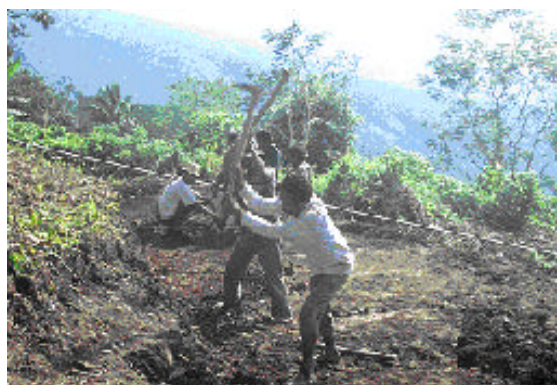
Building a road on top of the mountain. Liquiça District, East Timor © Francis Dobbs, World Bank.
