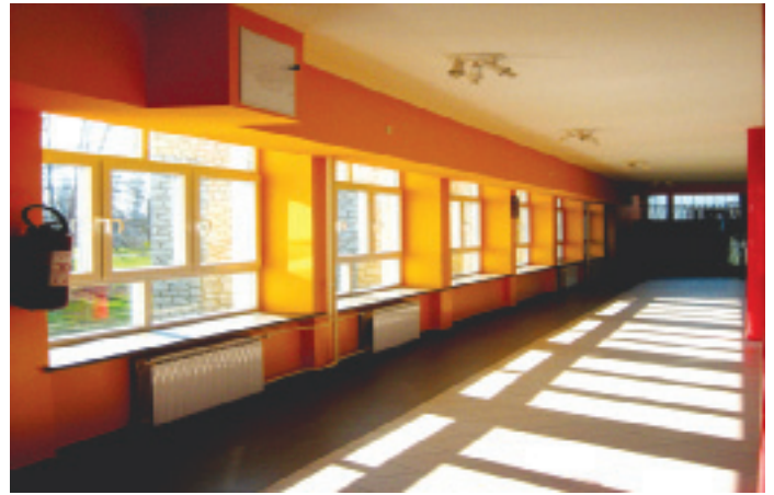
Replacement of wasteful light bulbs with new economical high-quality bulbs in a school in Karlovac
