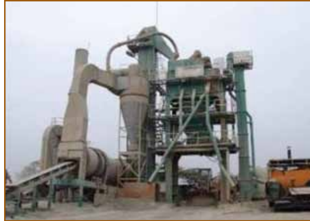
Modern Asphalt Plant near Hanoi, Vietnam
