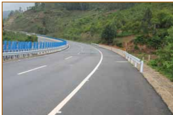
Four-Lane Expressway in Yunnan Province, China with Emergency Lane, Concrete Shoulders, and Concrete/Metallic Guardrail
