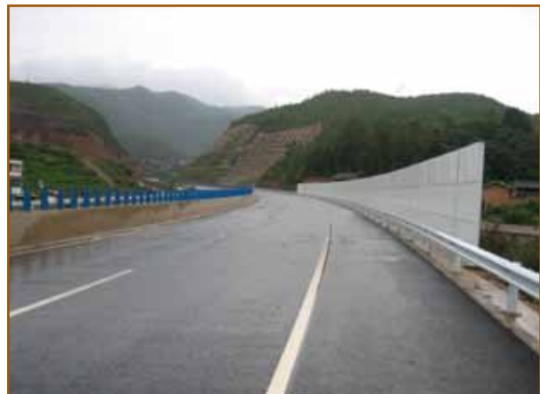
Expressway with a Mix of Concrete Crash Barriers in the Median Reservation and Metallic Crash Barriers on the Shoulders in China
