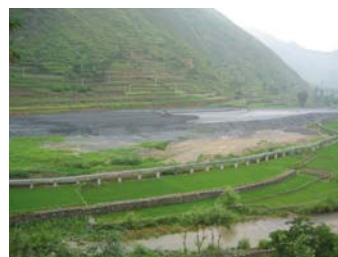
New Aqueduct Provided by Project
