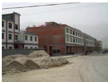
New homes for 15 resettled families in Wuyuping
