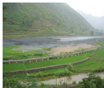
New aqueduct built by project
