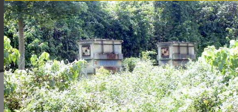
Switchyard Remains (Mt Coffee)
