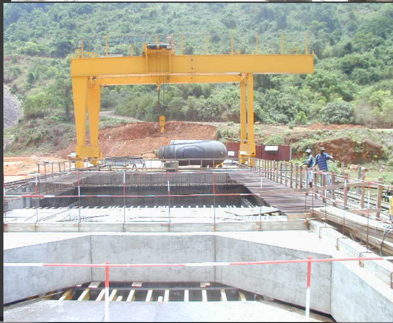
Construction of Bumbuna HEP, Sierra Leone
