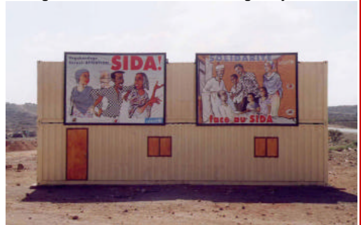
Figure: AIDS Posters on a building in Djibouti
