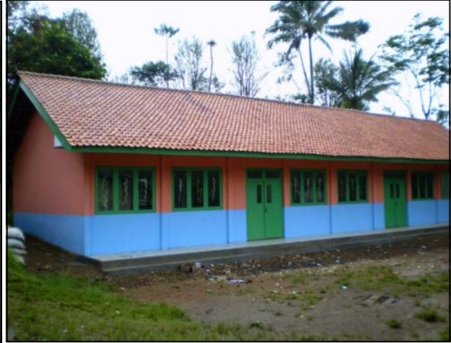
New school construction using PNPM Generasi funds.
