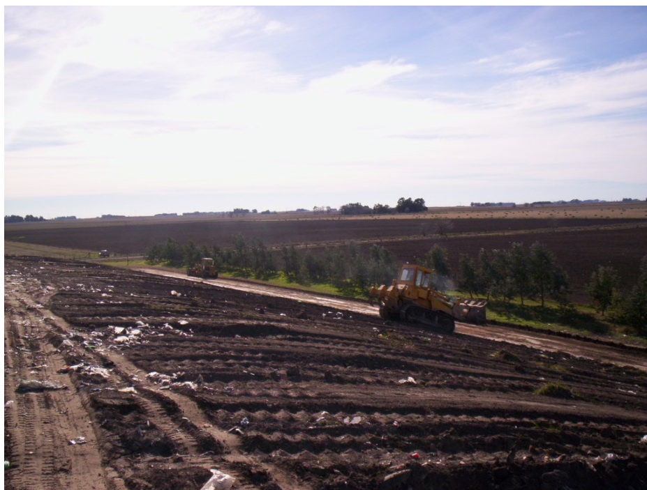
Figure 4. Cover works in Olavarría's landfill
