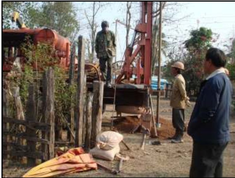
Figure 4. Drilling bore hole for domestic water supply
