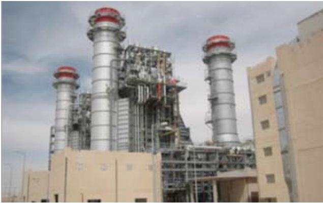
370 mega-watt combined-cycle Amman East Power Station – the first private power station in Jordan
