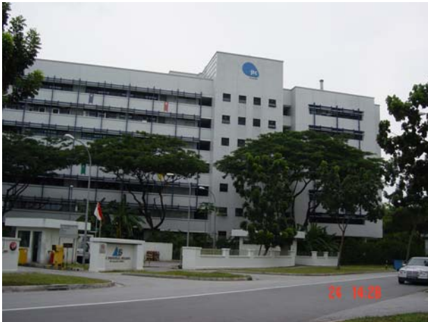
Figure 1: JTC ready built flatted factory
