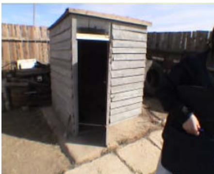
A typical latrine structure in Ulaanbaatar's Ger Area.
