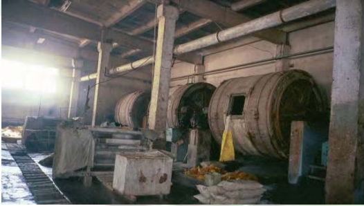
Belon Tannery, machines for tumbling skins with solutions. Wooden slats (lower left) are covering the open sewage line which channels the drained solution from these machines.
