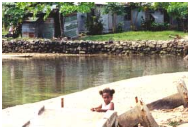
Figure 9. A Seawall in Qoma, Fiji
