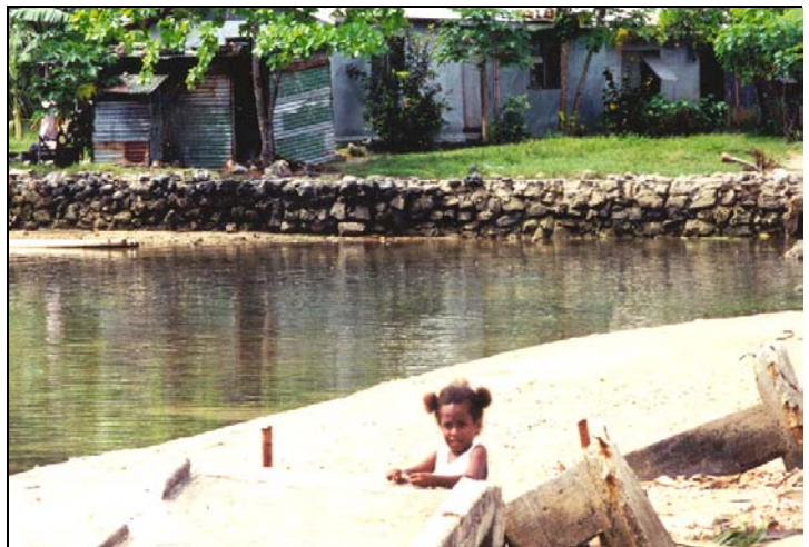
Sea walls are built throughout the Pacific to protect settlements against coastal erosion and storms. However, sea walls do not solve the underlying cause of erosion and may cause further problems downstream. In Qoma, Fiji (photo above) the community reported experiencing frequent inundation, which might have been exacerbated by their sea wall. Strategic replanting of mangroves might well have been a more efficient solution to guard against periodic inundation.
