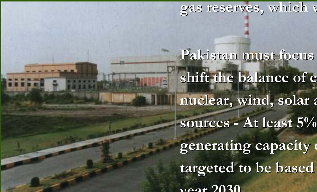
CHASNUPP Power Plant
