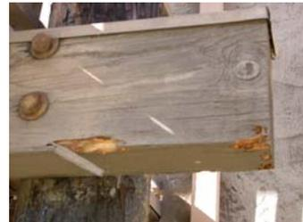
Photo: 26 - Drywood termite damage,
