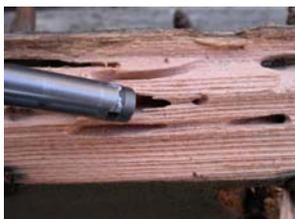
Photo: 27 - Drywood termite damage,
