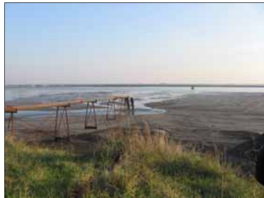
Fly ash landfill at the Nikola Tesla B TPP
