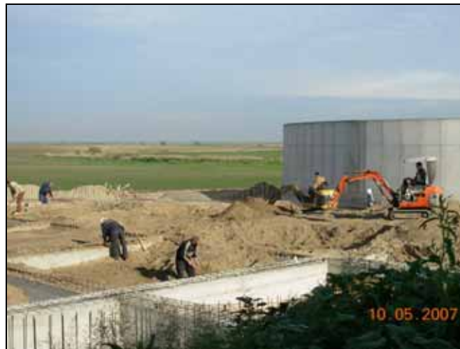
Construction of manure storage facilities on Napredak Farm (Novi Sad, May 2007)
