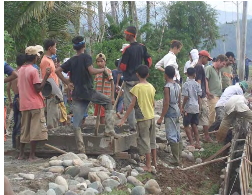
community work to build their own road in Tiro, Pidie, Aceh
