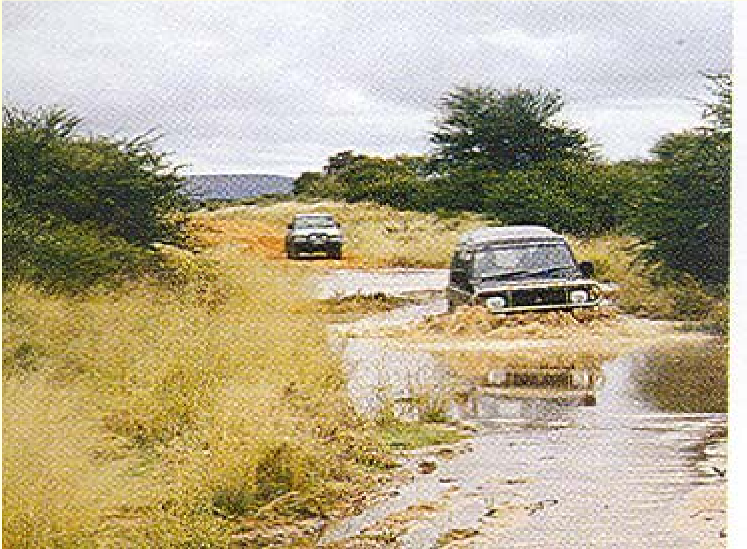
Short sections of road in poor condition can benefit significantly from spot improvement works.
