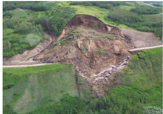
Figure 1. Translational landslide, Beatton River Valley, British Columbia, Canada, 2001.
