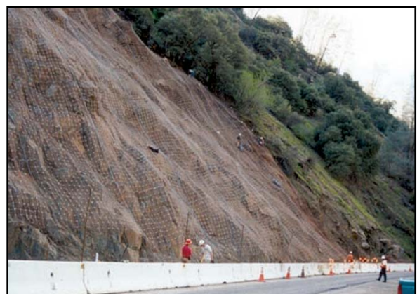
Figure 5. Protective wire mesh (net) over rock adjacent to road
