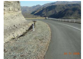
Road after improvement
