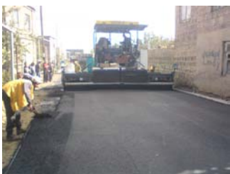
Road Construction Work
