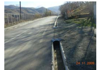
Road after improvement
