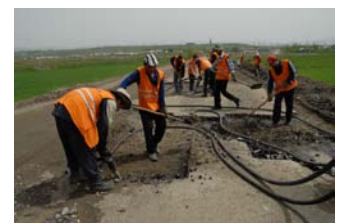
Road construction work
