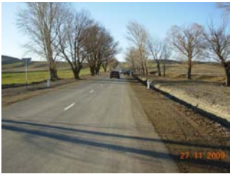
Road after improvement
