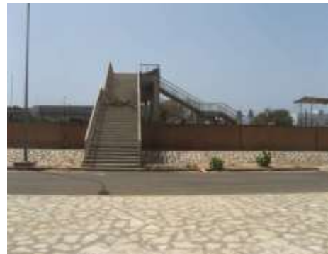
Non accessible footbridge
