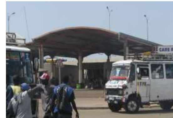
Bus station building is not accessible
