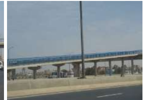
Footbridge with a ramp ( strong slope and absence of resting zone)
