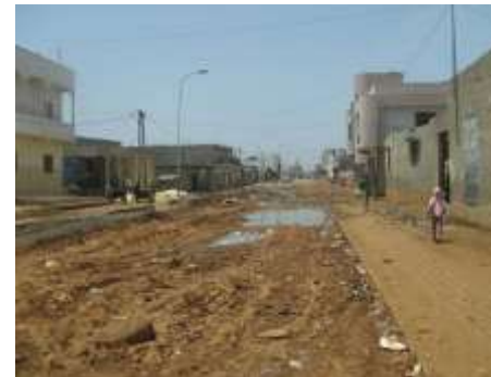
Road in very bad state
