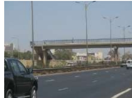
Footbridge with stairs
