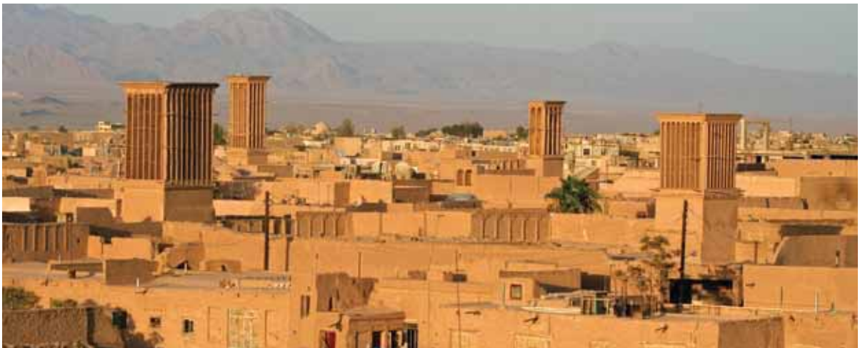
FIG. 14 > Badghirs, or traditional Persian wind-towers, used to cool down buildings in Yazd (Iran)
