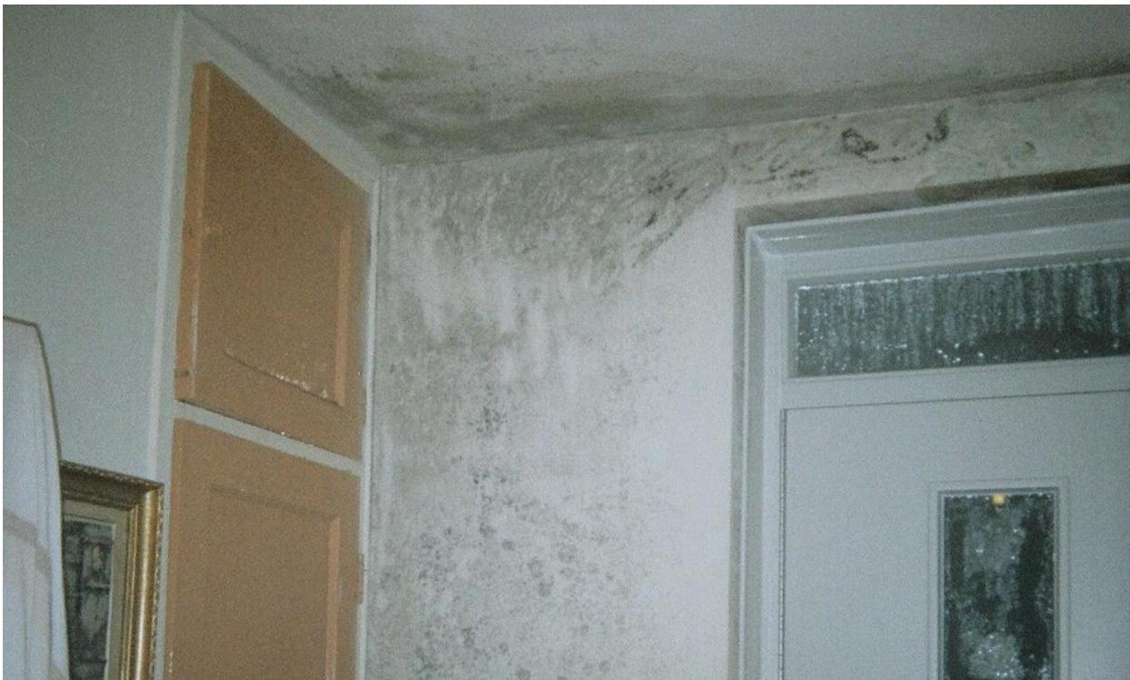
*Figure no. 3: Tidy on the outside, mouldy on the inside. Walls in the entry hall of Claire's recently refurbished flat. Source: Claire/SCIBE*
