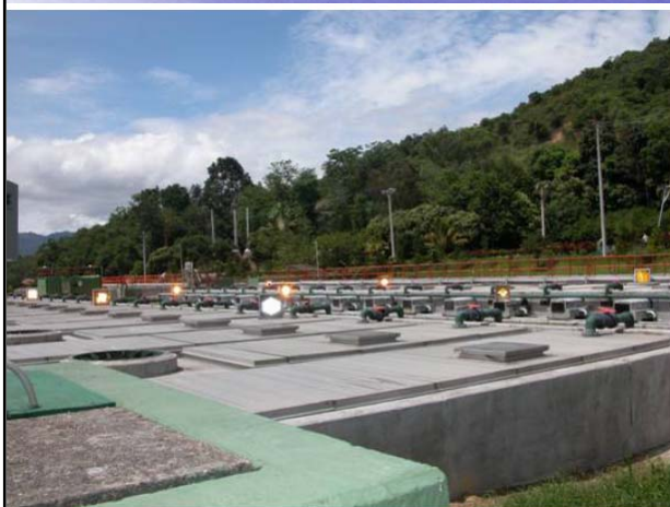
Figure 6. HRPM Configuration Used at the UASB Reactor Area
