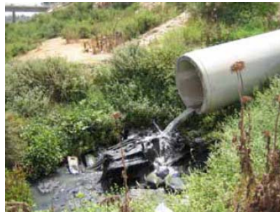
Figure 2: Municipality of Khenichet: Sewage is discharged into the river
