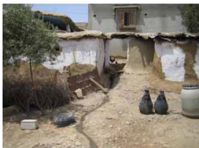
Figure 3: Doaur of Chtauoma: Grey water is discharged from homes into the street.
