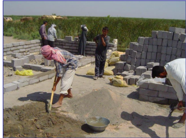
The establishment of brick-making factories provided income, employment and building materials (UNHCR partner)
