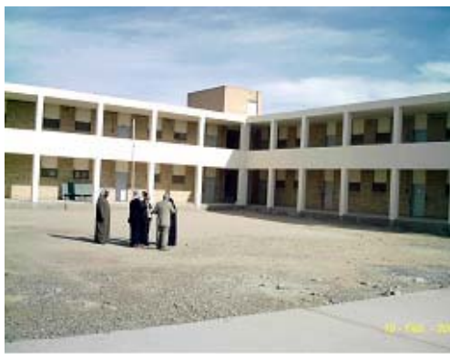
School yard of the newly constructed Al-Ameer Secondary School in Najaf
