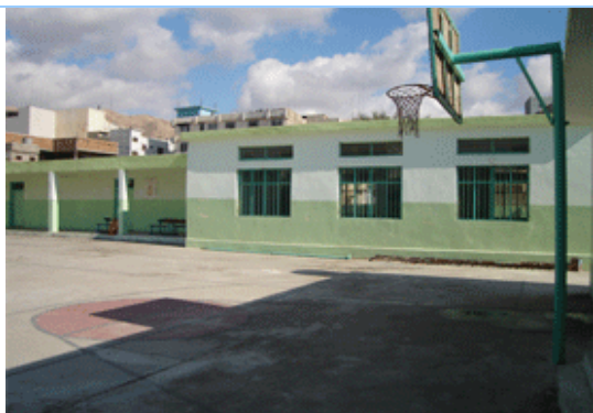
School yard of a newly constructed Secondary School in Baghdad (ESCRP Project) (May 06)
