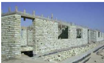
School construction in Najaf
