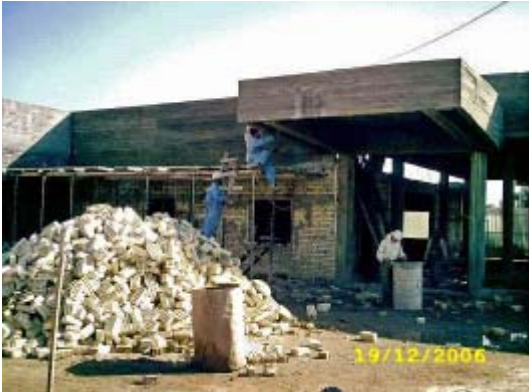
Hospital Renovation in Sadr City
