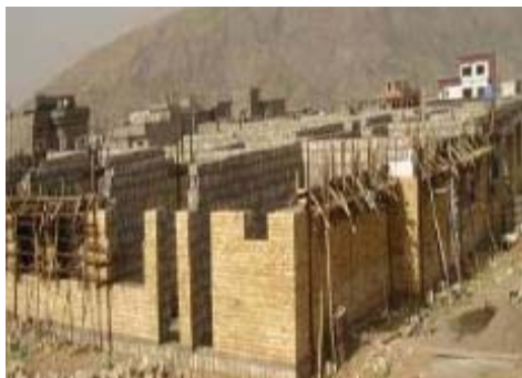
School Construction in Derbandy Khan/ Sulaimaniyah (April 2007)
