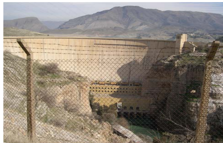
Dokan and Derbandikhan Hydropower Facility
