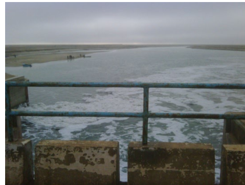
NAS Kok-Aral Dyke and Spillway in November 2010
