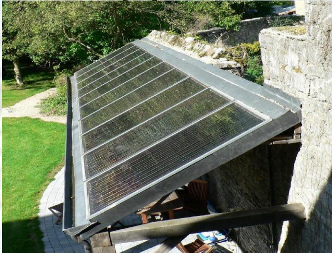
Conventional PV Solar for Residential Water Heating
